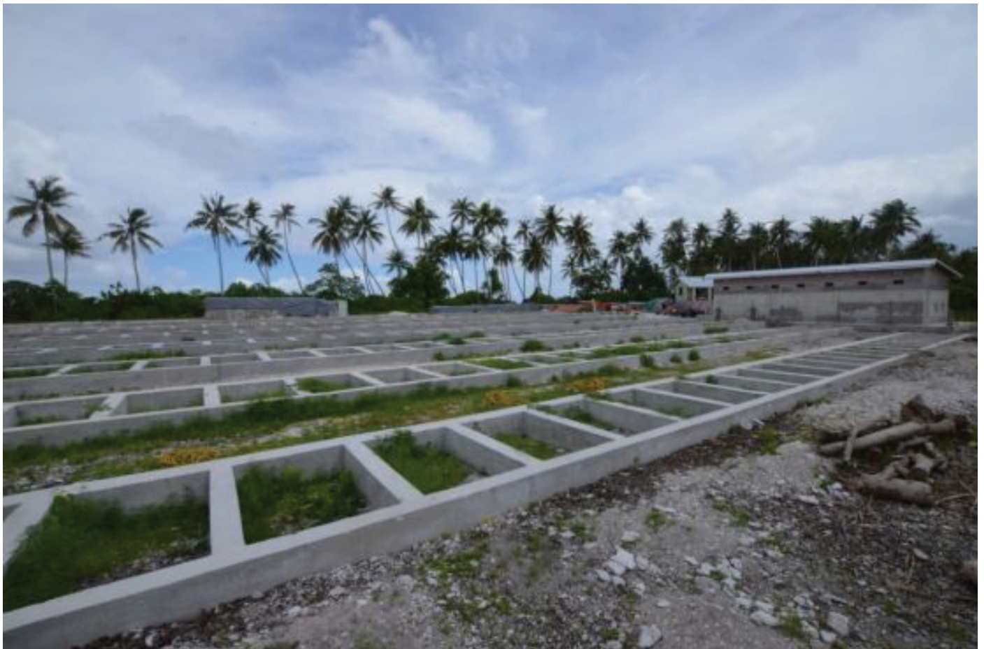
Nukunonu array foundation with inverter/battery building and generator shed in background (Power Smart Solar photo)
